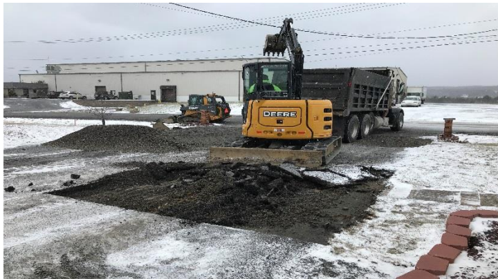
Digging out the bad spots in the front section
