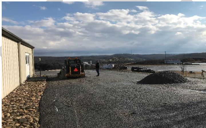
Rear Section under Construction
